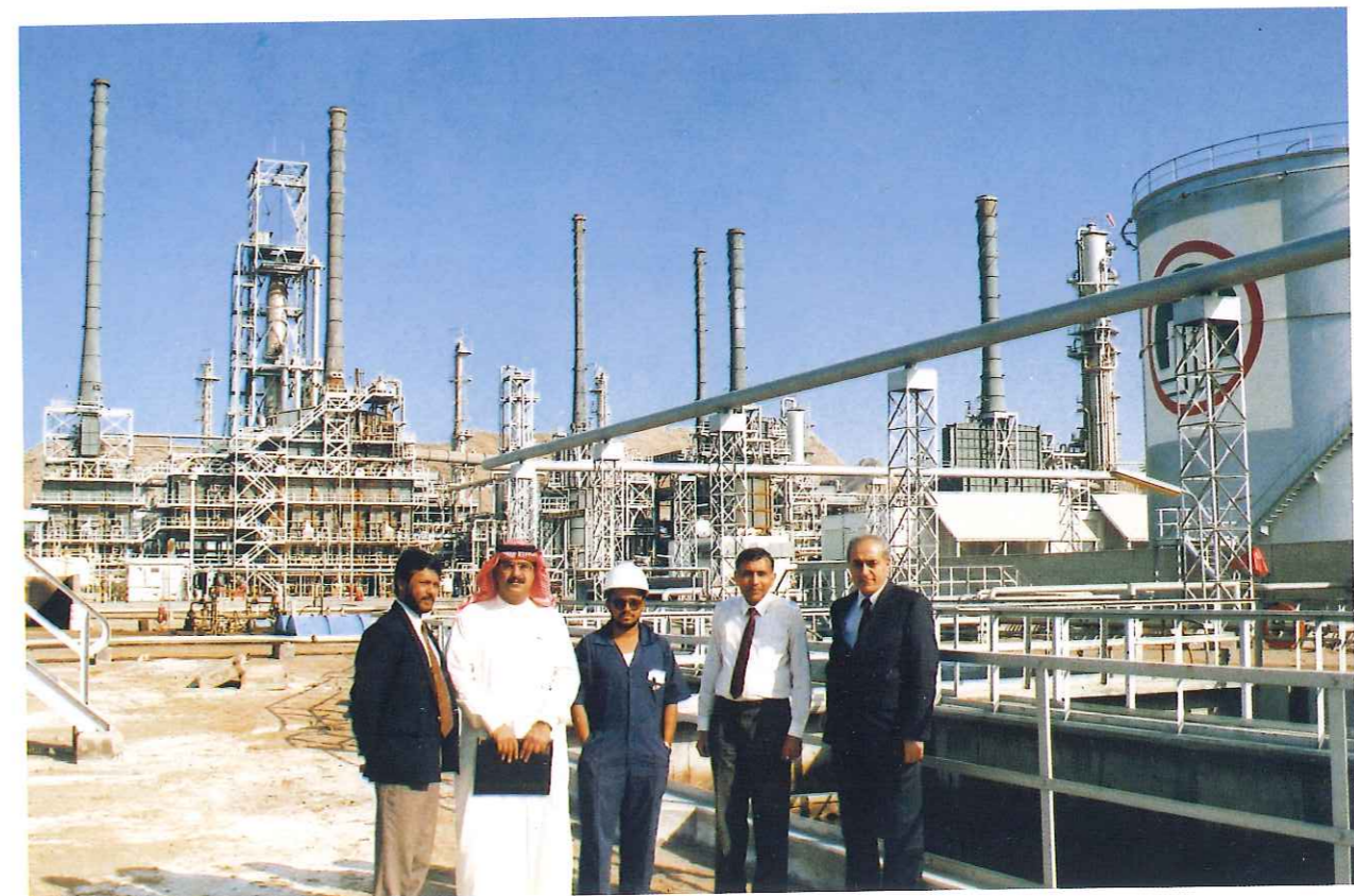
Unleaded Gasoline Production - Mina Al Fahal
